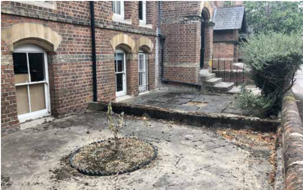
Poor quality impermeable patterned concrete surface to No.10
