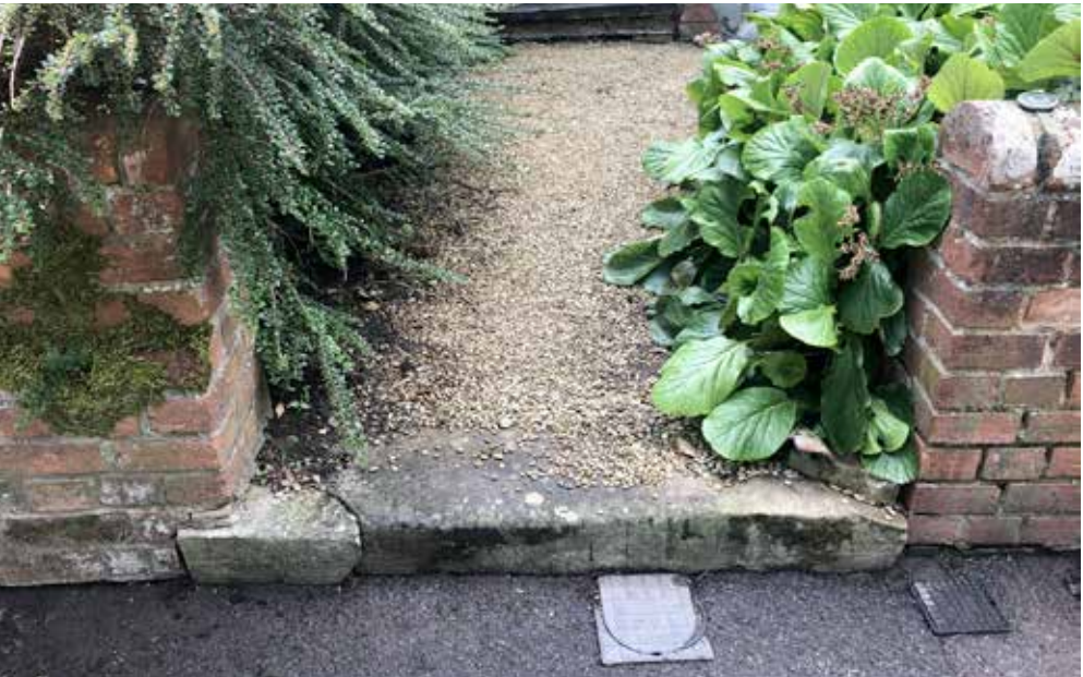
Damage to original step and new gravel path at No.8
