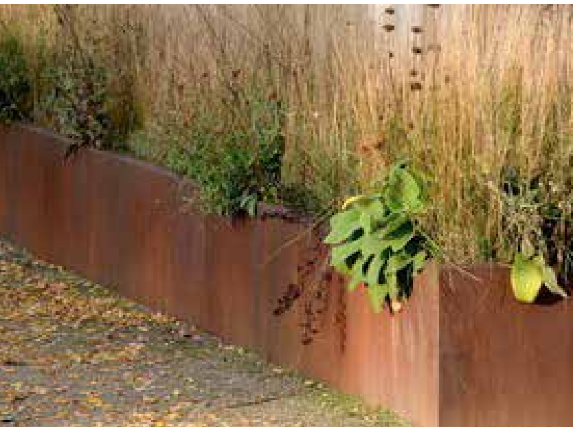
Rainwater from new roofs irrigate plants in troughs, reducing the rate of run off in to the mains system.
