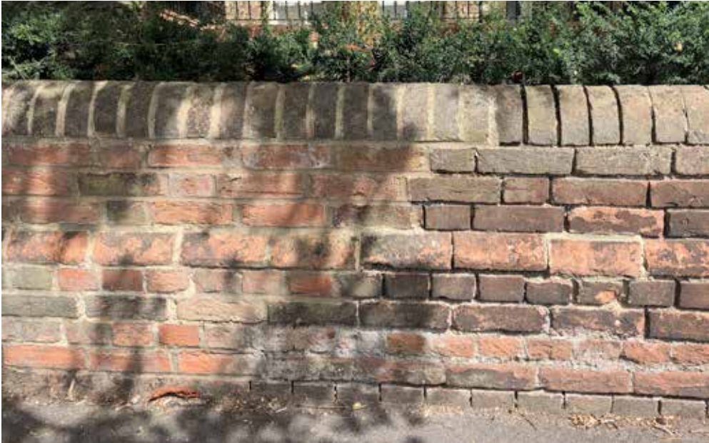
Existing low vernacular walls in need of re-pointing repairs
