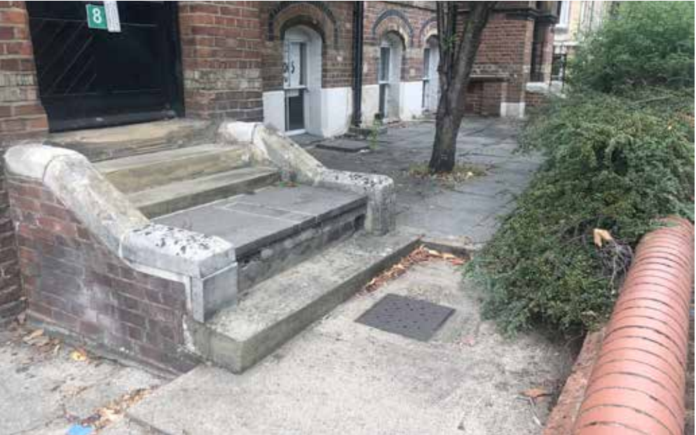
Original steps repaired with poor quality concrete tread at No.8
