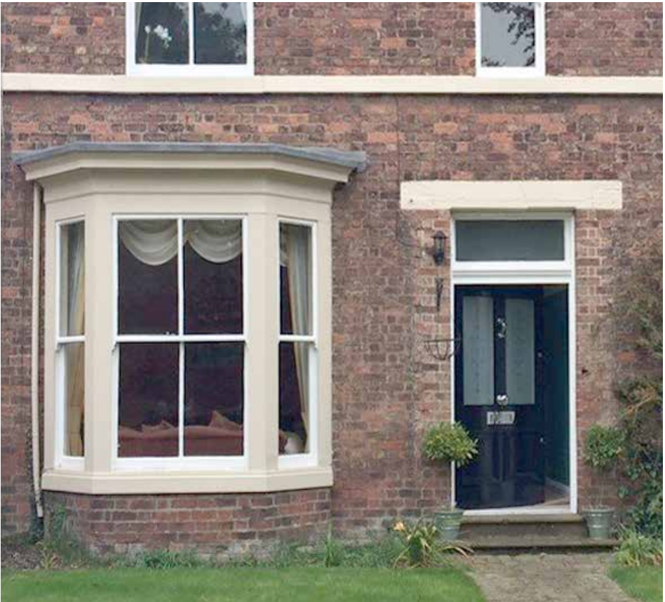
Whilst most of the building performance upgrades will be internal, replacement double glazing can improve thermal performance greatly whilst being almost indistinguishable from the existing.
