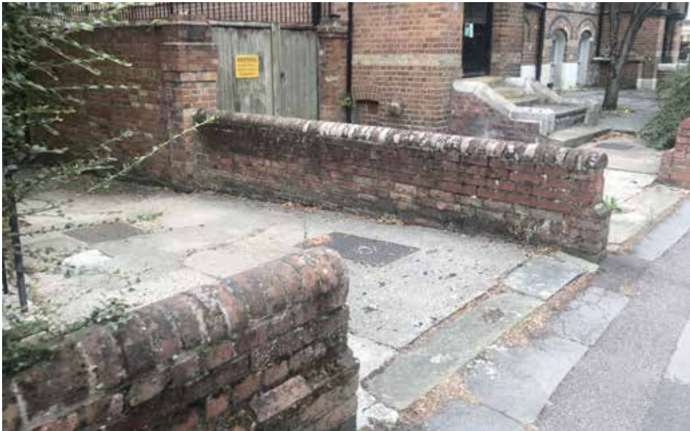
Original yorkstone edge with poor quality concrete parking at No.9
