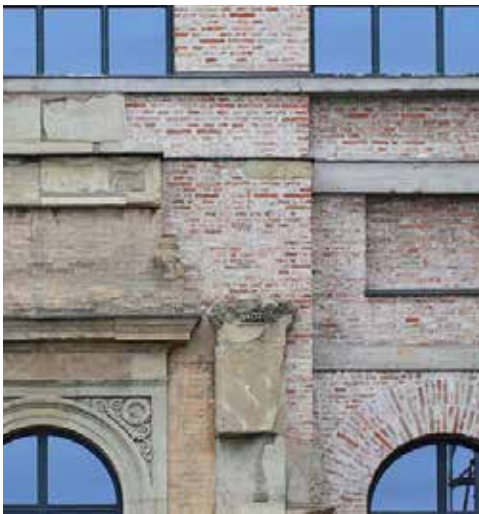
Contemporary repair interwoven with historic brickwork
