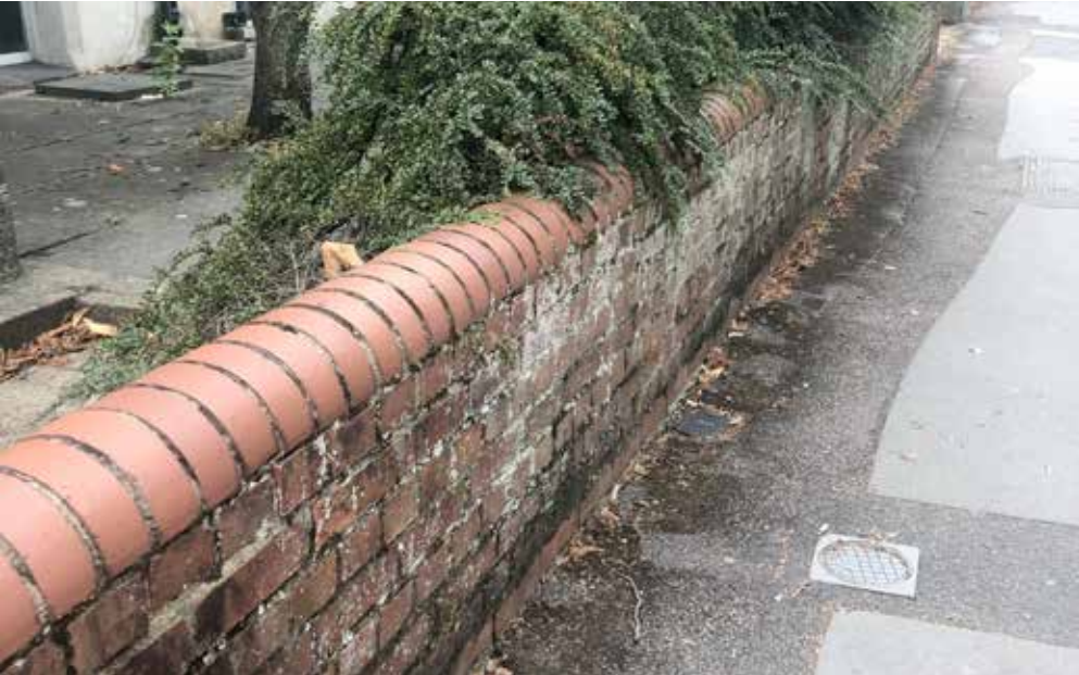
Inappropriate brick selection for bullnose coping repair at No. 8
