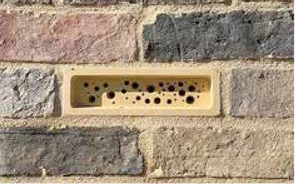
Integrated brick bee houses
