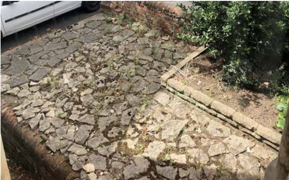
Poor quality crazy concrete paving and walls to No.5 & 6
